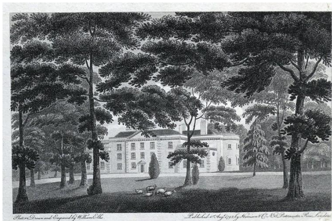
Figure 34. This drawing and engraving produced by William Ellis (London: Harrison & Co., 1792), shows Streatham Park.
